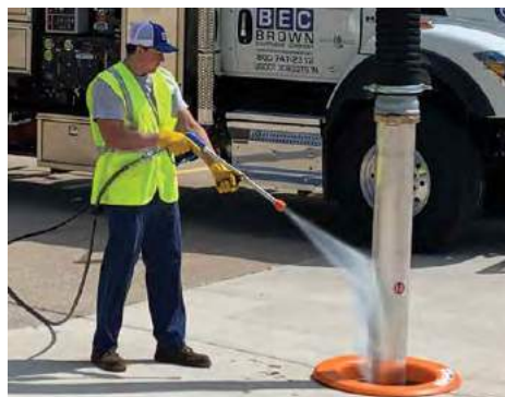
The spray system also provides the water volume, cleaning, and killing power required for effective SSO clean up.
